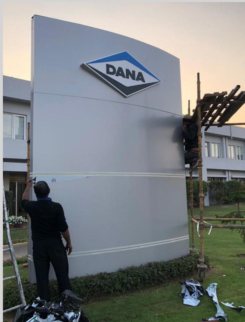
ACP Totem with Poly Board on MS Structure
