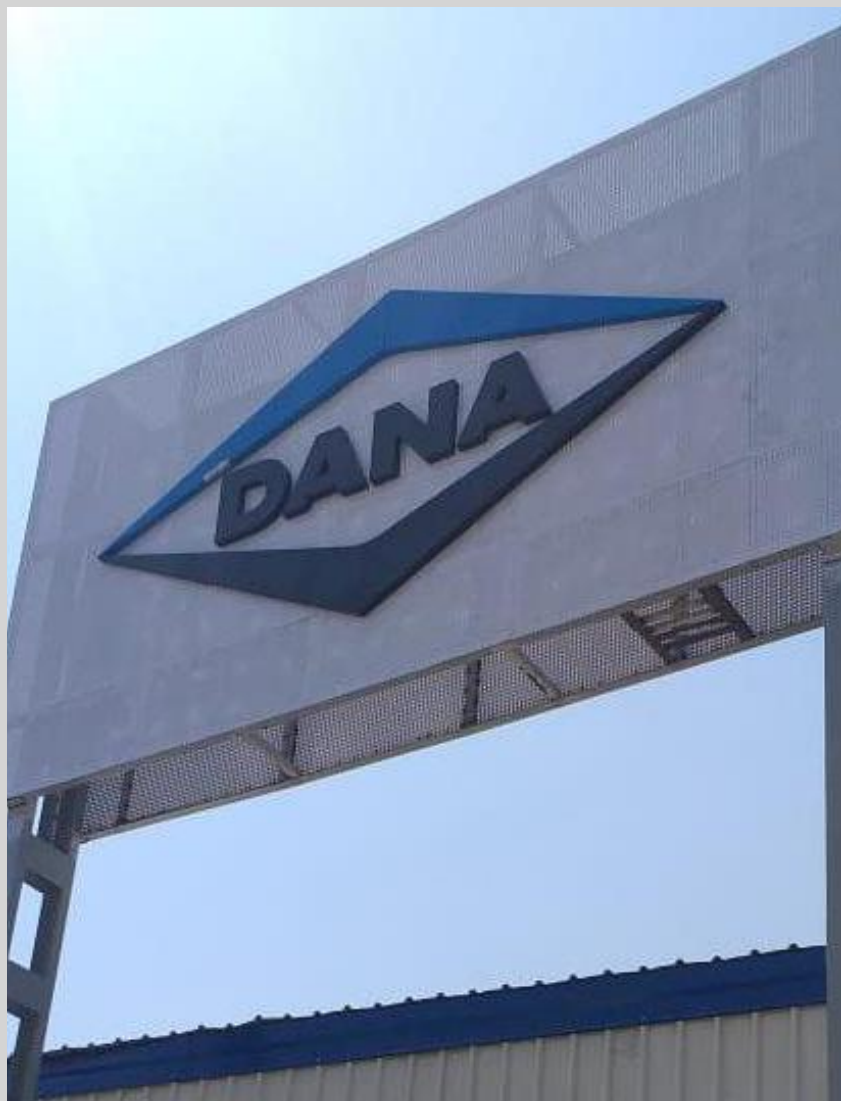
Structural Signage: SS Powder Coated Letter on MS Sheet
